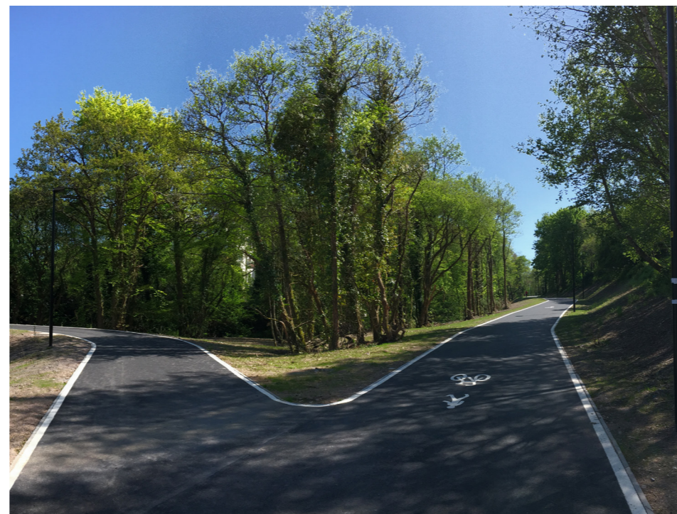
Figure 3.3 - View of the existing greenway to the west of the site
